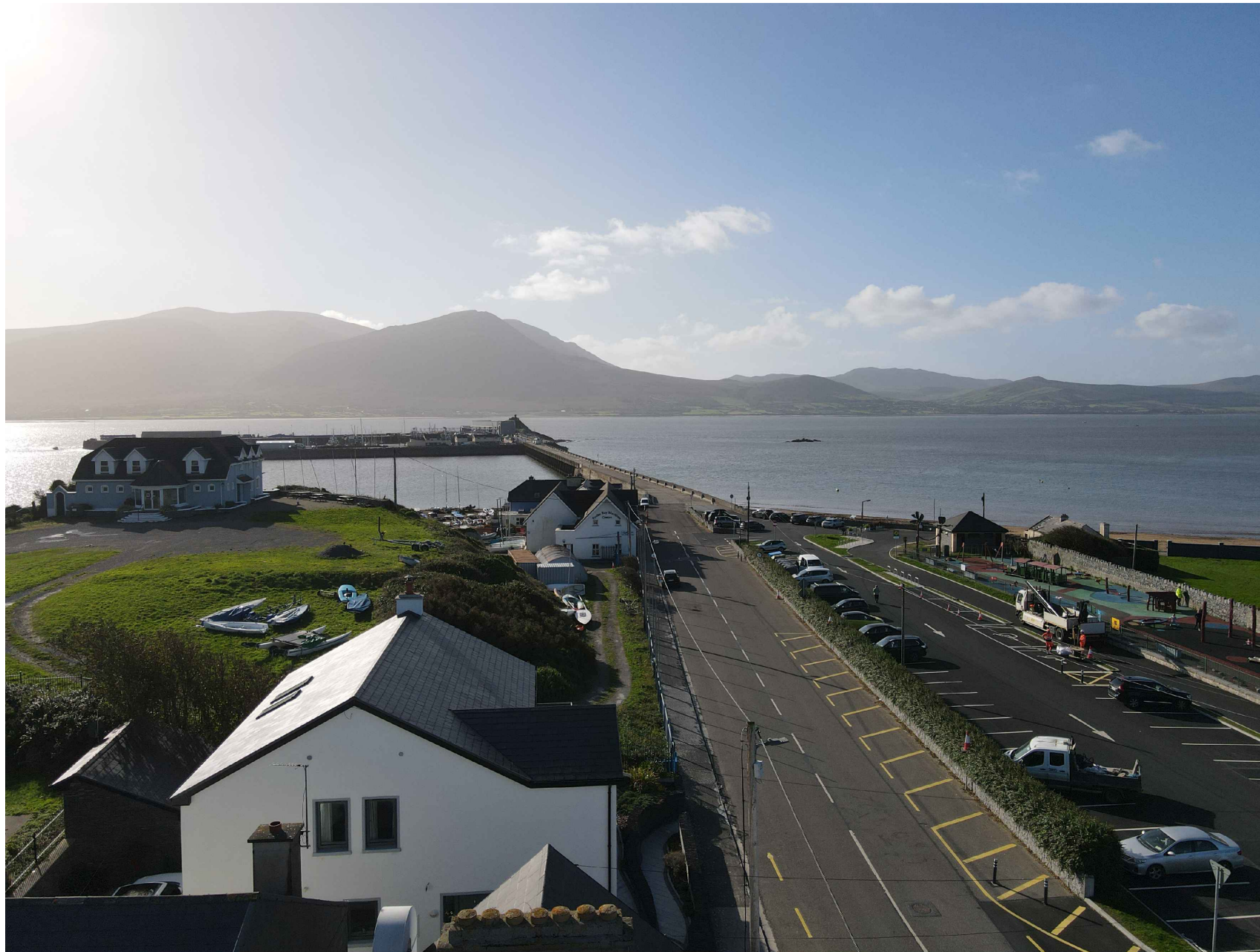
Existing Aerial View 2 Scale NTS
