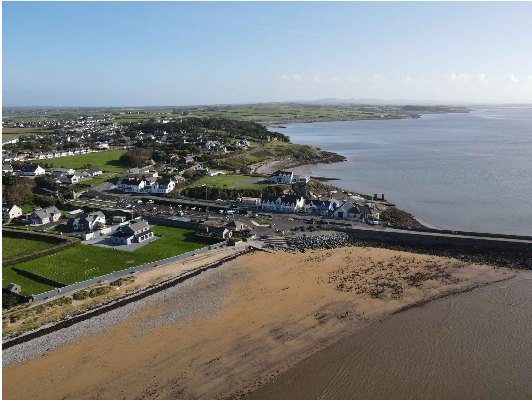
Existing Aerial View 3 Scale NTS
