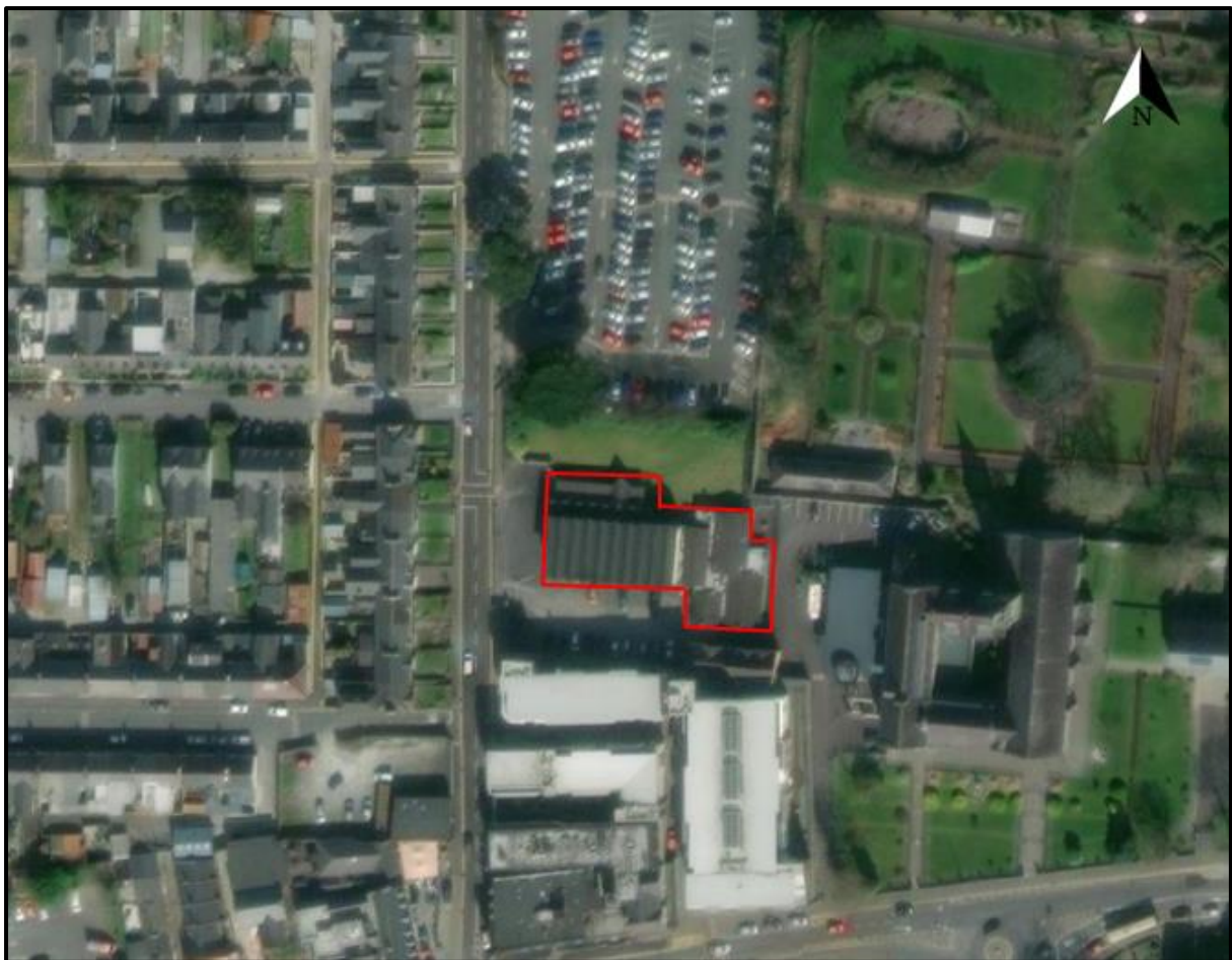
Figure 2. Aerial image showing the structure to be demolished (Red).
