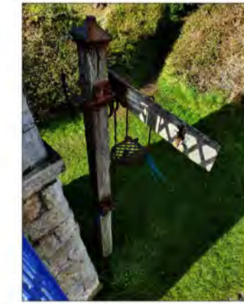
B. RAILWAY SIGNAL POST
