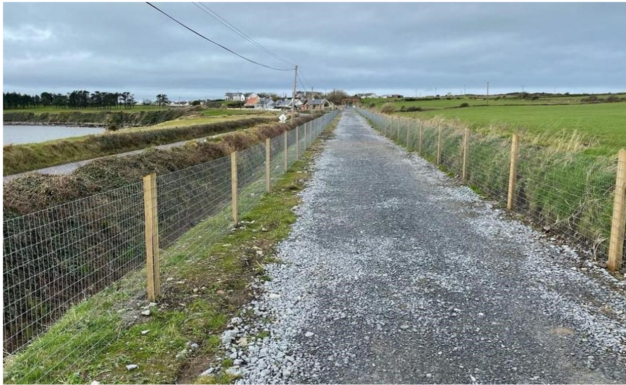
Fencing along the Greenway
