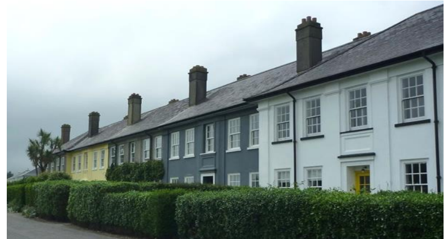
Figure 3.96: View of Cable Station Terrace
